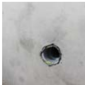
BELOW GRADE SIDE CONDUIT FOR WIRING INTAKE.
